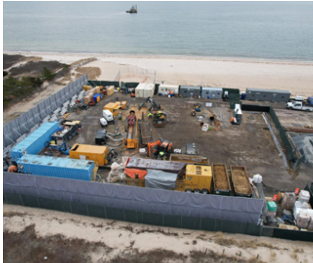
Example shore crossing work site
