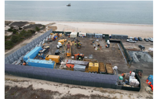
Example shore crossing work site
