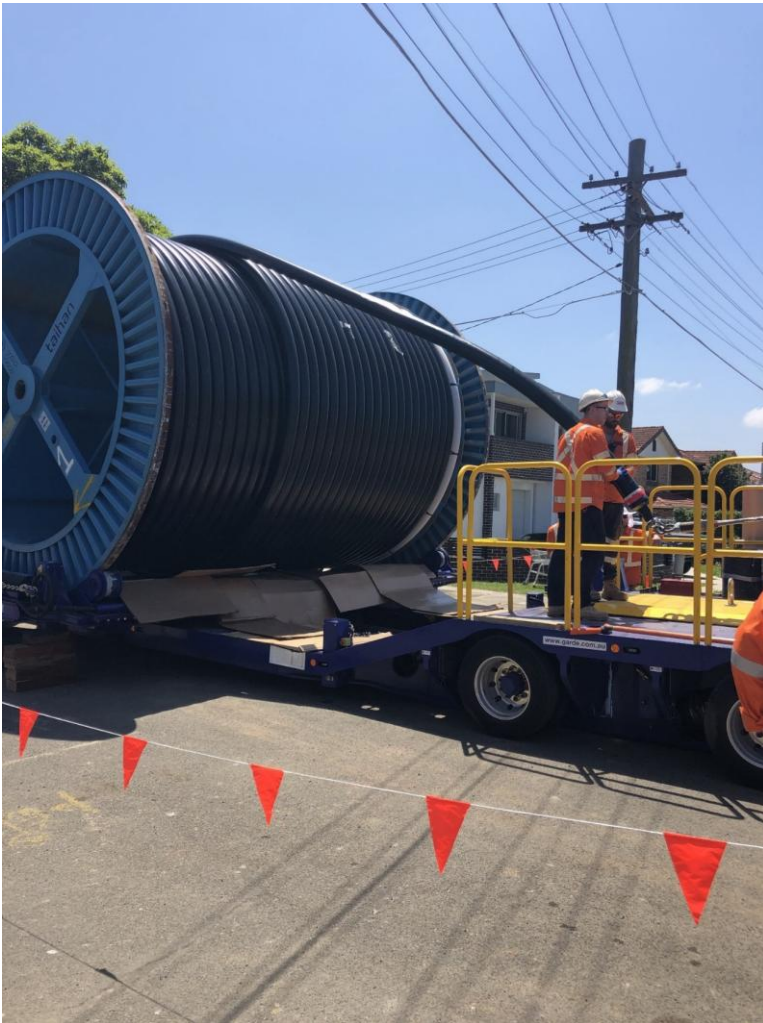
Figure 4-28 Cable being fed from a cable spool into conduit (Australia)
