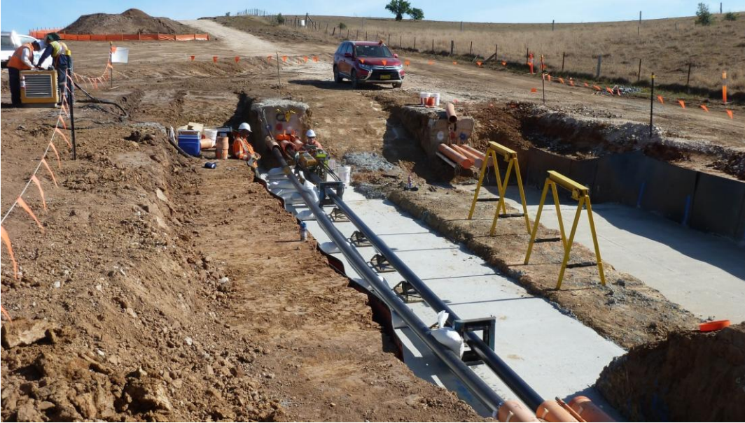
Figure 4-29 Example of a caterpillar pit (Australia)
