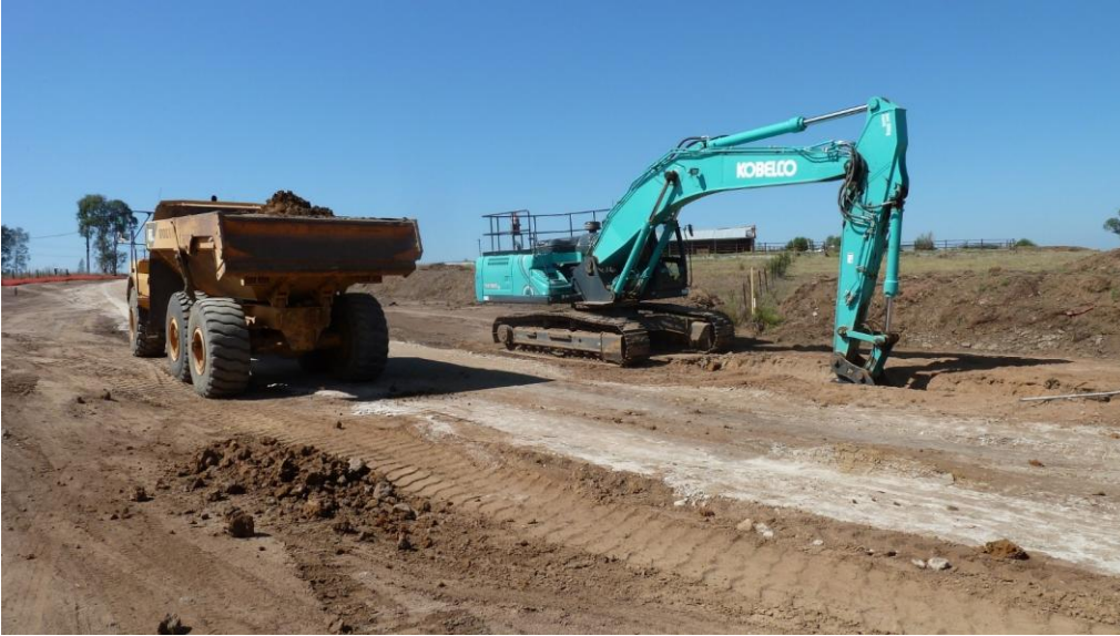
Figure 4-25 Cable trench excavation (Australia)
