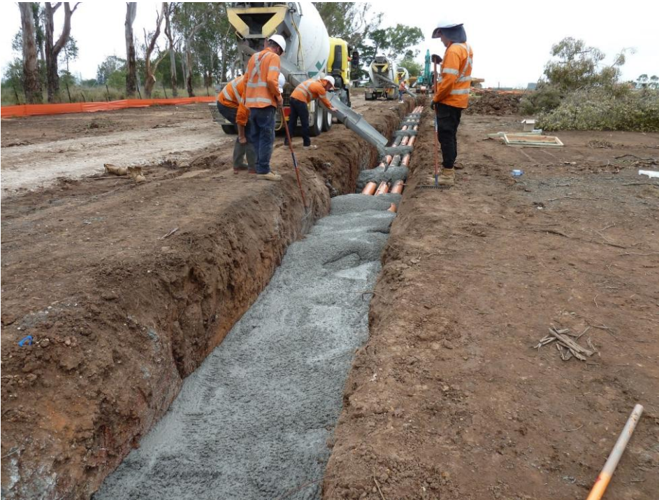
Figure 4-27 Thermal fill installation (Australia)
