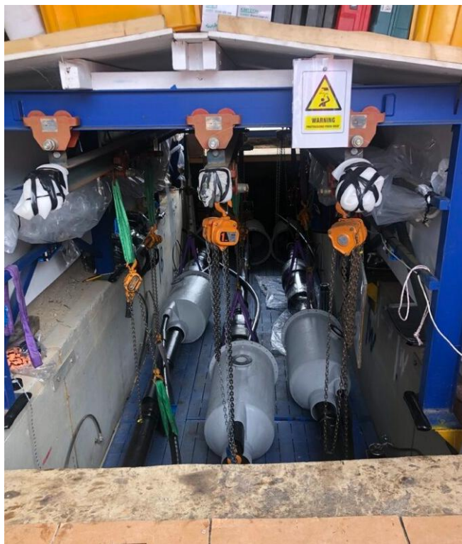
Figure 4-22 Cable jointing underway in a controlled environment (Australia)
