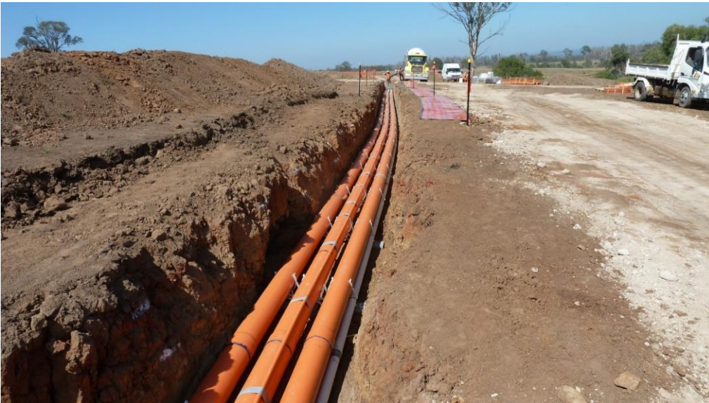
Figure 4-26 Installation of conduit in a trench
