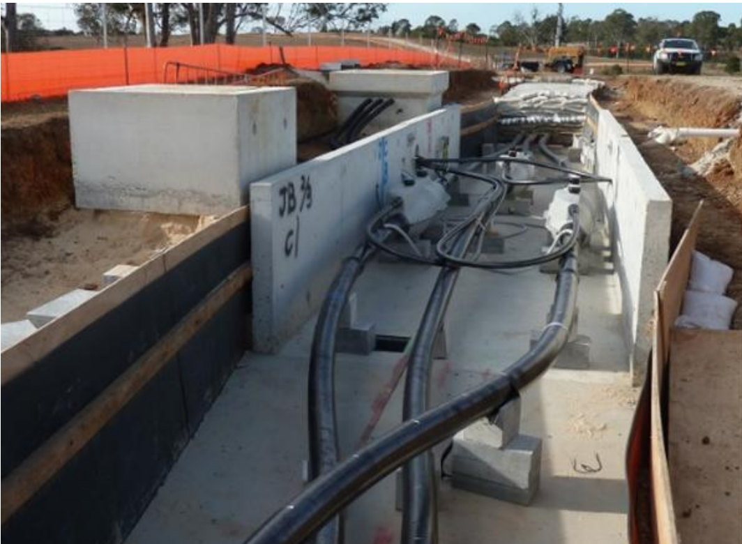
Figure 4-30 Joint bay ready for backfill (Australia)
