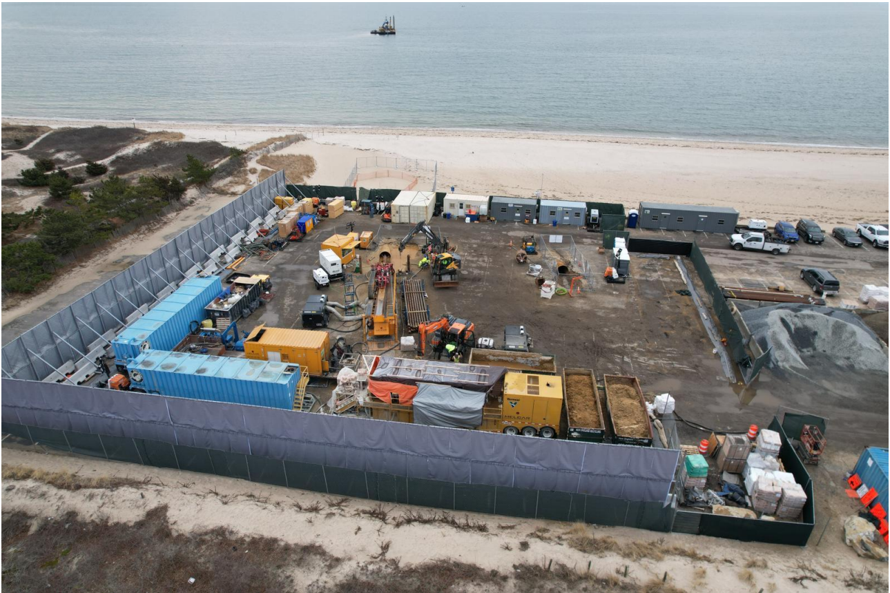
Figure 4-12 Shore crossing drilling operation, Vinyard Wind USA
