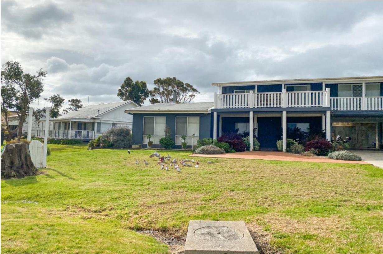
Figure 22-9 Typical view of LCA 5
