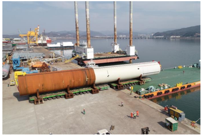
Self-Propelled Modular Transporters (SPMT) moving a monopile from a transport barge on the Jeonnam project
