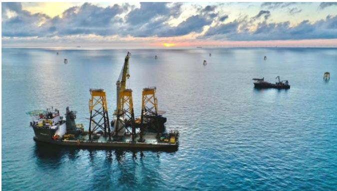
Bokalift 1 installing jackets at Changfang and Xidao Offshore Wind Project
