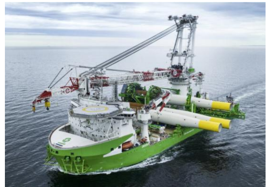
Orion installing monopiles at Vineyard Wind
