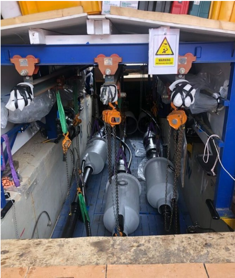
Figure 4-35 Cable jointing underway in a controlled environment (Australia)
