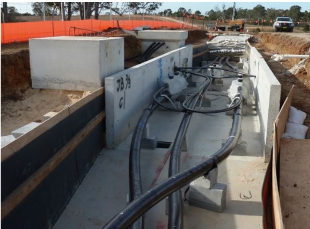
Figure 4-43 Joint bay ready for backfill (Australia)
