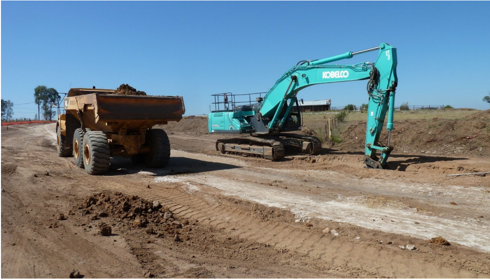
Figure 4-38 Cable trench excavation (Australia)
