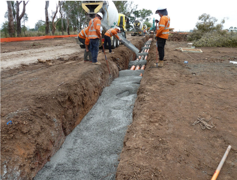
Figure 4-40 Thermal fill installation (Australia)
