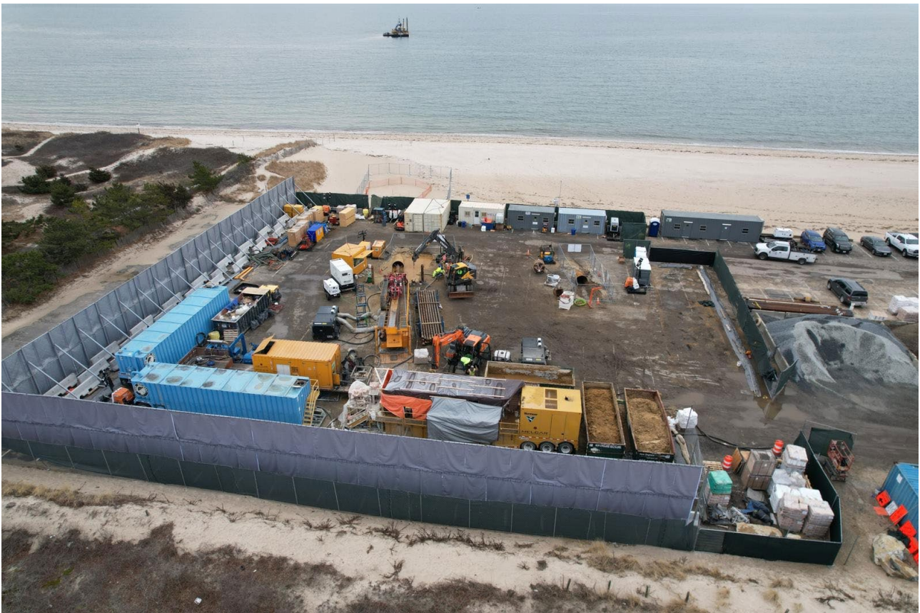
Figure 4-25 Shore crossing drilling operation, Vinyard Wind USA
