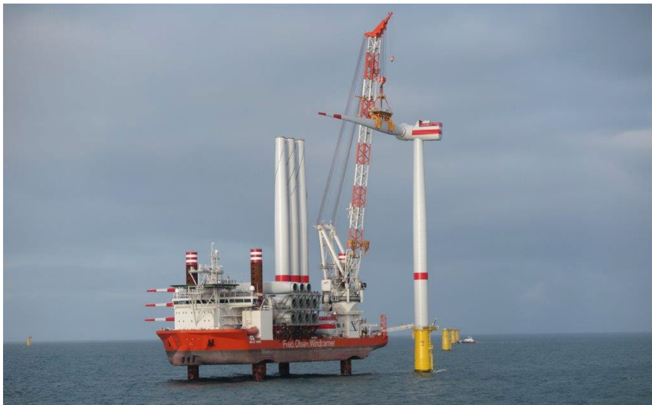
Figure 4-14 Offshore wind turbine installation via jack-up vessel
