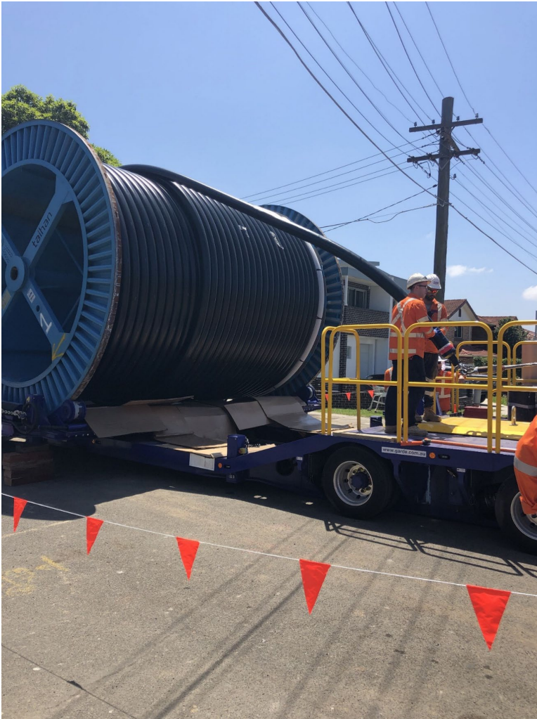
Figure 4-41 Cable being fed from a cable spool into conduit (Australia)
