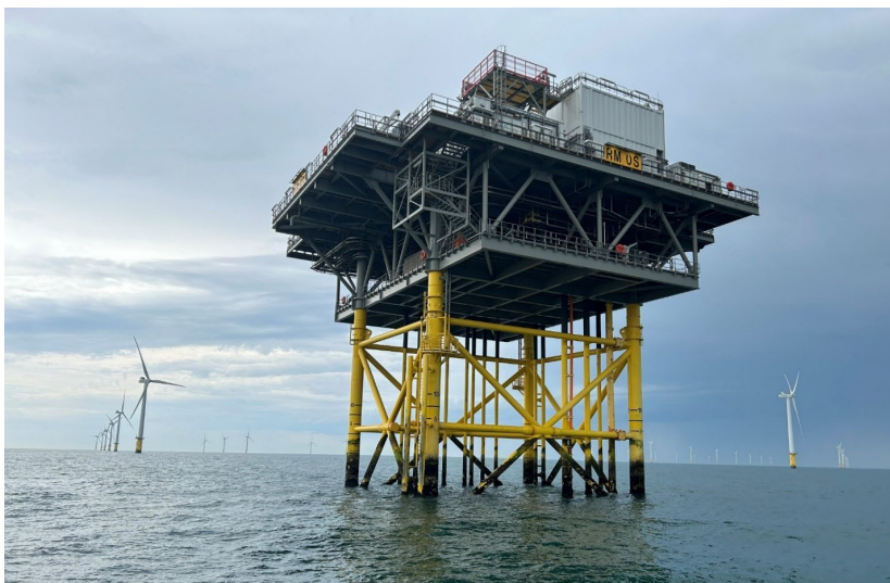
Figure 4-9 Piled jacket foundation for an offshore substation
