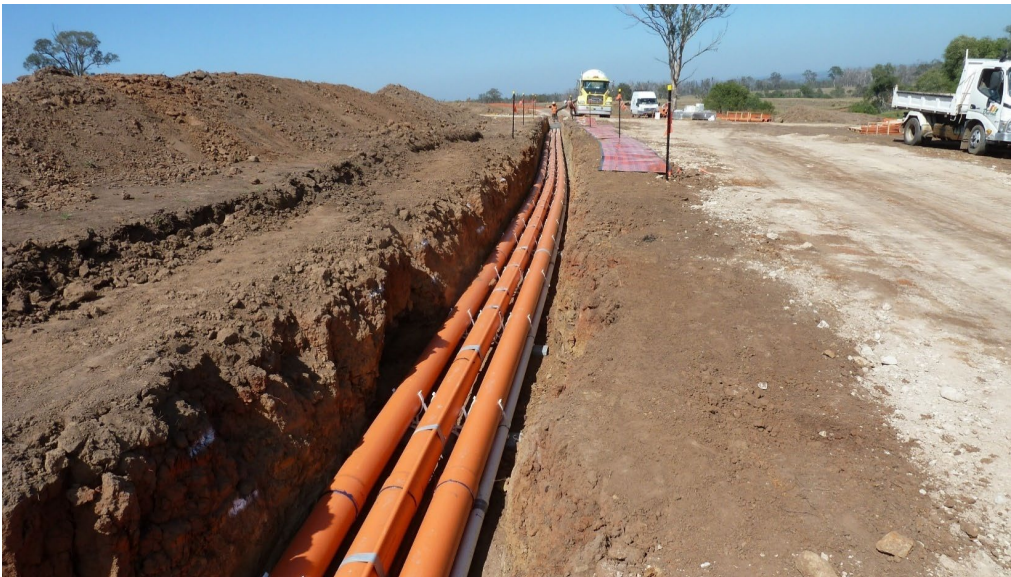
Figure 4-39 Installation of conduit in a trench
