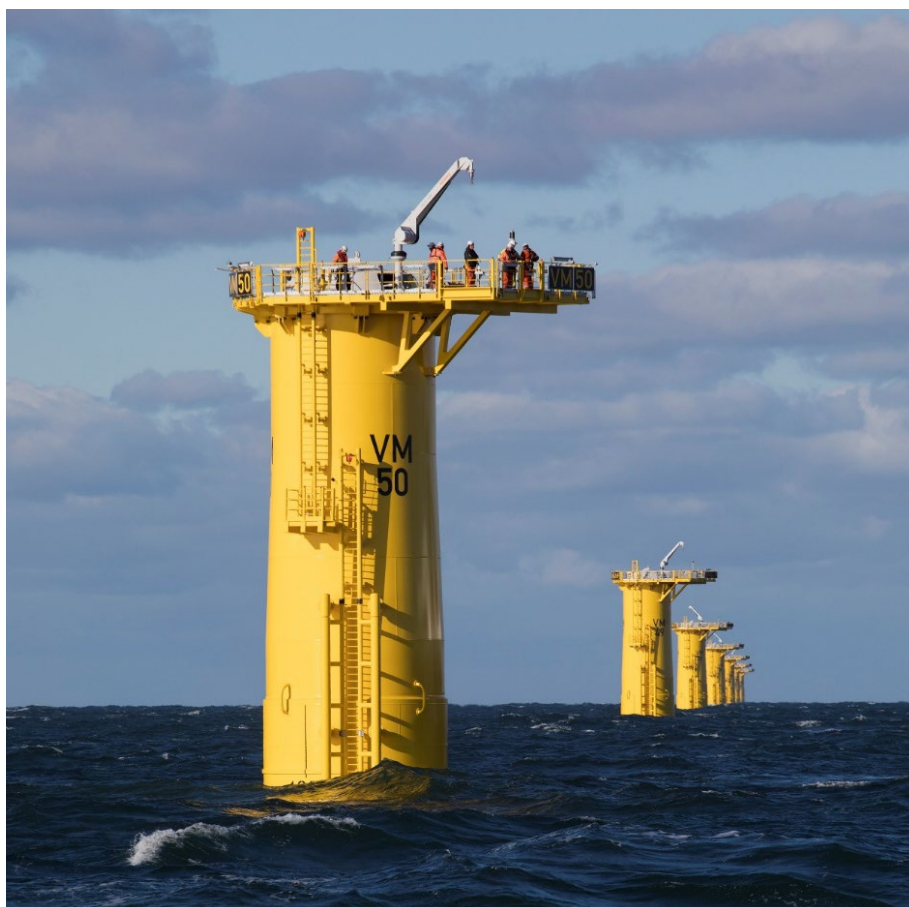
Figure 4-8 Transition piece ready for turbine installation
