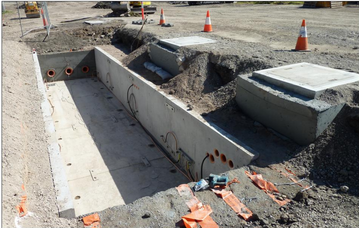
Figure 9-1 Example of joint bay prefabricated liner
