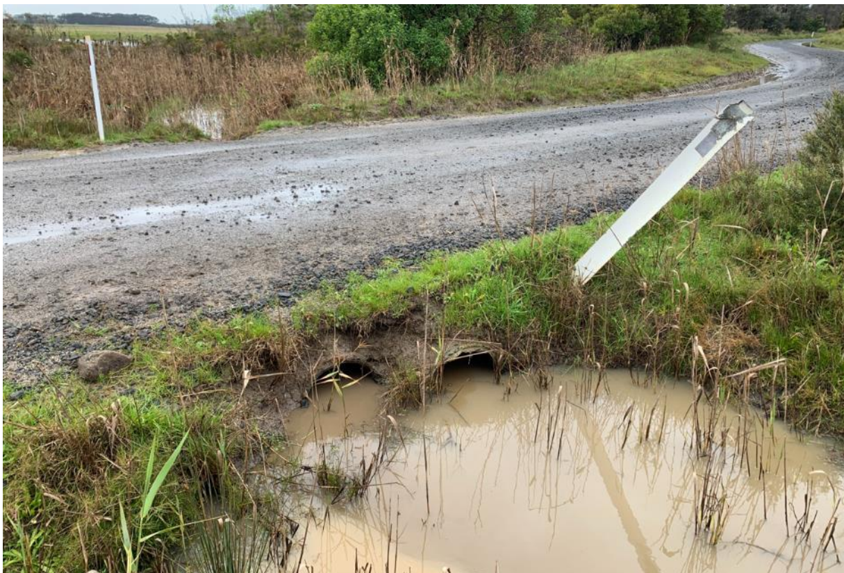
Figure 7-6 Piped culverts crossing under Reeves Beach Road (looking north) (Photo taken 14/07/2021)
