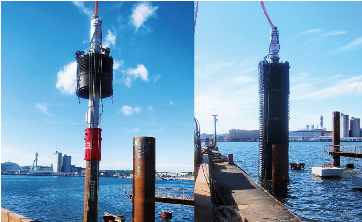
Figure 13-1 Example noise reduction bellows ( www.ihciqip.com )
