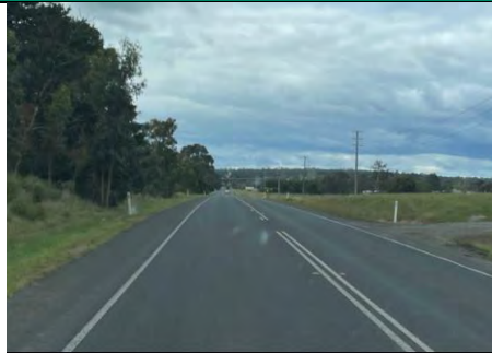
Firmins Lane – looking eastbound
