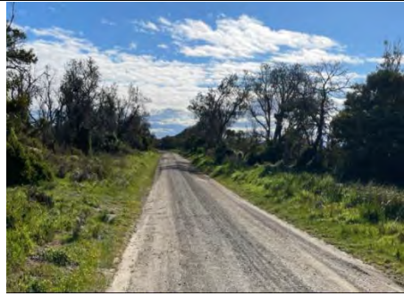
Reeves Beach Road – looking westbound
