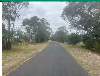
Giffard West Road – looking eastbound
