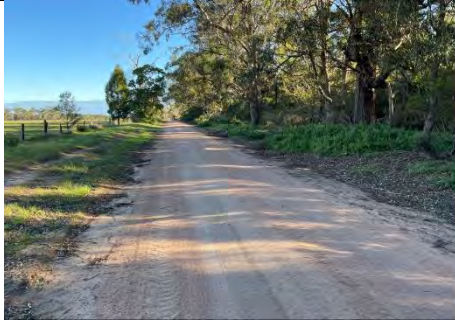
Stringy Bark Lane – looking southbound
