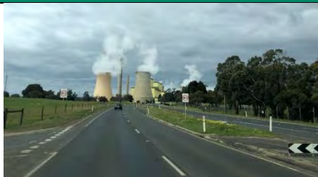
Hyland Highway – looking eastbound
