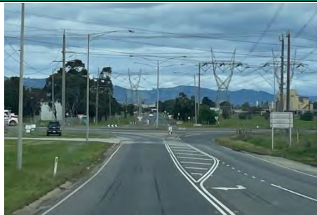
Tramway Road – looking southbound
