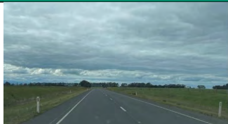
Hyland Highway – looking eastbound
