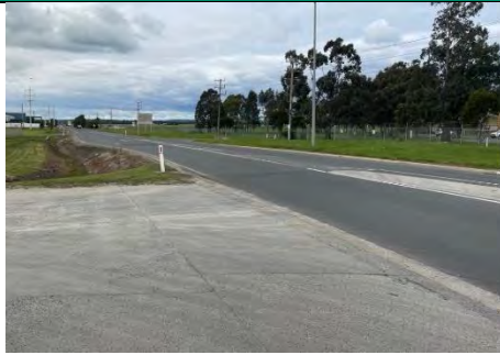
Firmins Lane – looking eastbound
