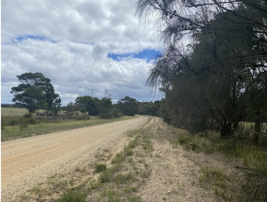
Figure 10-8 Curve restricting sight distance at Giffard West Road (east) looking north-west (Source: AECOM, 2025)
