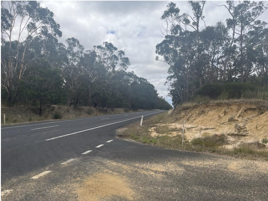
Figure 10-9 Crest restricting sight distance at Four Mile Creek Road looking north onto South Gippsland Highway (Source: AECOM, 2025)
